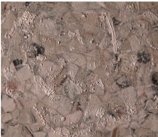
Figure 4: Disinfectant residue on vinyl flooring.
