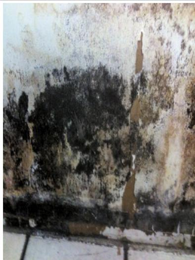
Figure 1: Water damaged wall covered with mold.
